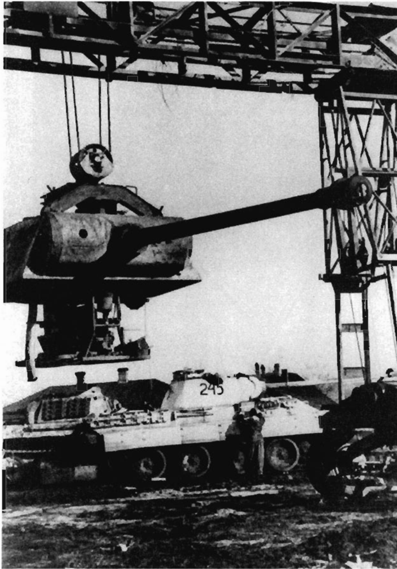
The gantry crane was developed for heavy loads. However, setting it up took more than an hour.
