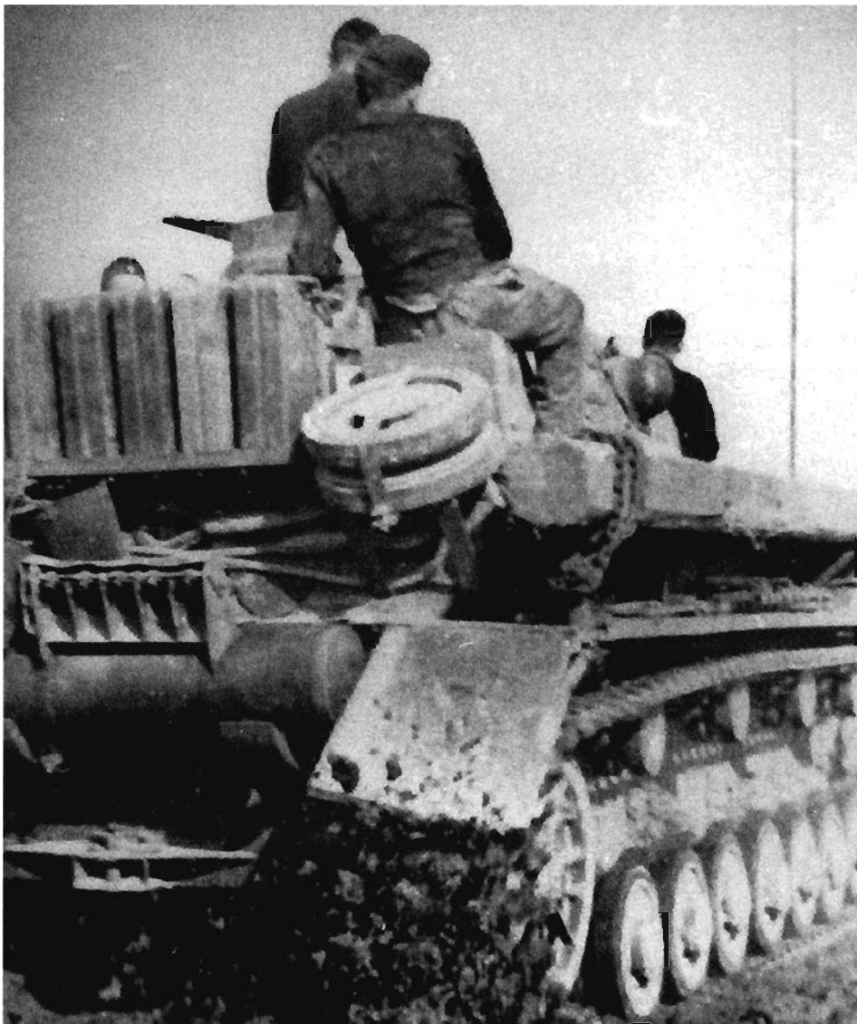
In the Second World War, the limited driving range of the predominantly gasoline-fueled tanks was a particular problem. The practice of carrying additional cans of fuel on the rear deck or roof of the turret was risky but frequently necessary.
