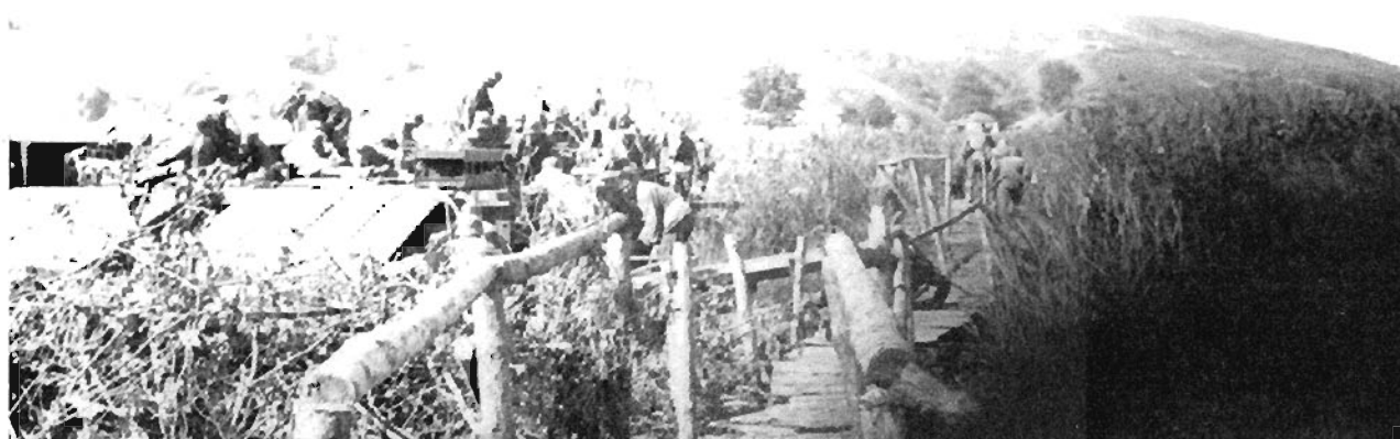
So-called infantry (assault) bridges are generally built next to the tank crossings.
